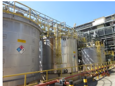
Stripped wastewater tank
